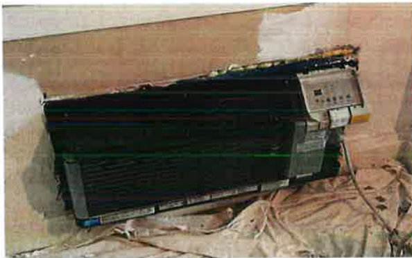
Unoperational PTAC and Spot Cooler
