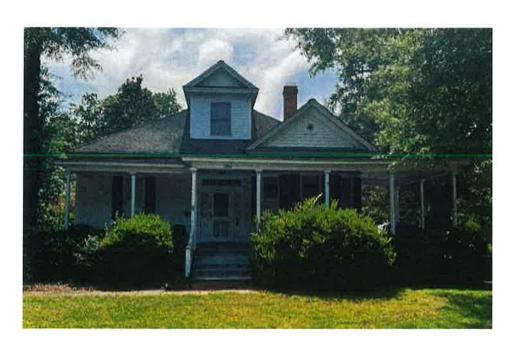
Porch roof is very shallow. Shingles are not the best roofing option. Have leaks currently with shingled roof. Urgent repairs needed.
