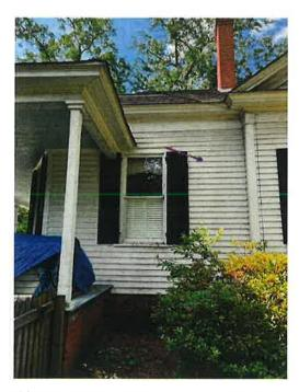
Water runs off porch roof onto top of window and onto Gas Meter (behind bush). Foundation remains damp in this area.
