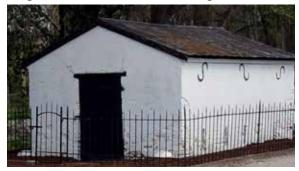
to assist in the ventilation and to keep the powder dry. It also features anchor plates known as earthquake bolts. These plates are connected to a tie rod or bolt which provides structural reinforcement to the masonry structure.
