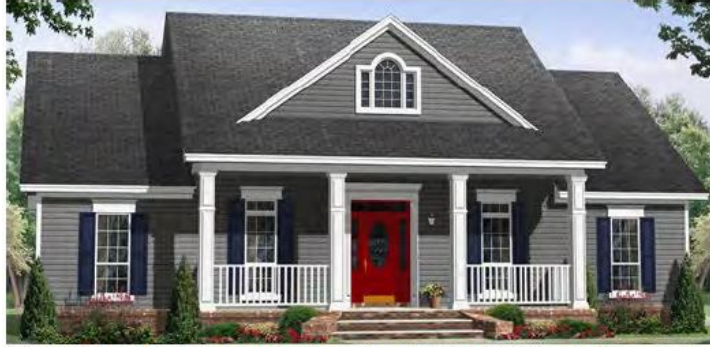
This house has a slab foundation that is raised an average of 18 inches from the ground, and the foundation is clad with brick.
