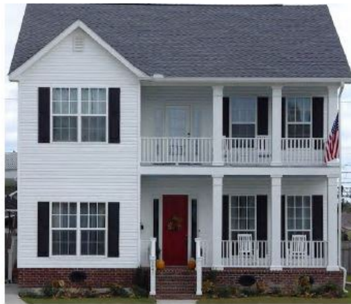
Example of residence with an 18-inch crawl space clad in brick.
