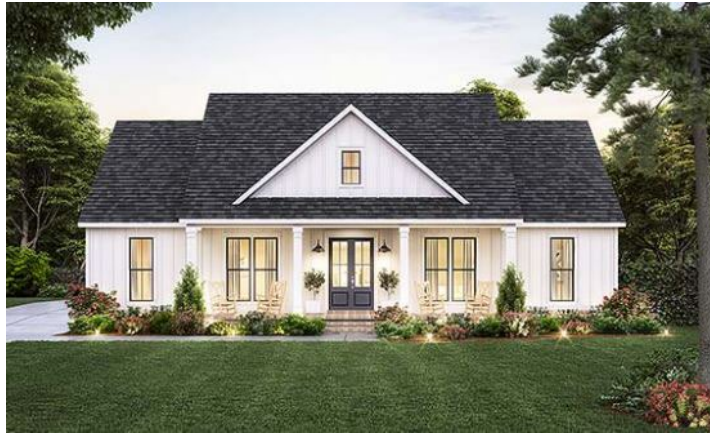
This residence has a slab on grade foundation, and the first 18 inches from the ground are clad in brick.
