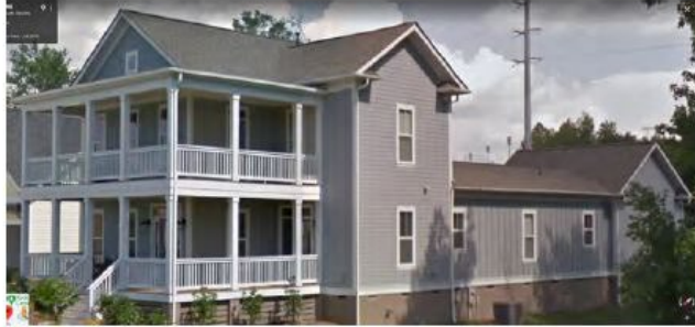
This house has multiple windows, a wrap-around porch, and façade line changes through different roof styles and number of stories on the side.
