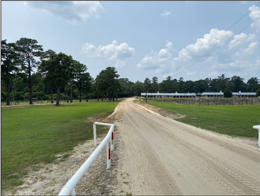
Photograph 3: A northwestern facing photograph of the equine facilities in the middle portion of the site.
