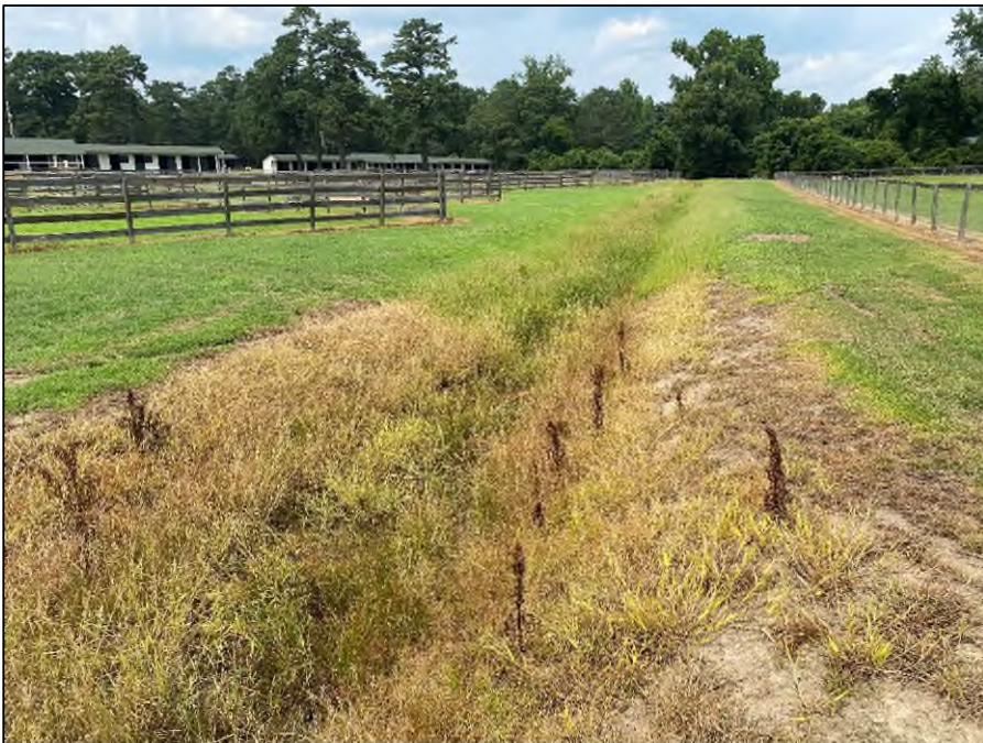
Photograph 16: A representative photograph an excavated ditch facing northeast.
