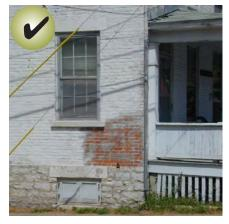
Perform a test patch to determine that the cleaning method will cause no damage to the material surface.
