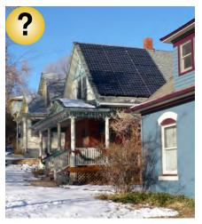
Minimize the visual impacts of skylights and other rooftop devices. It is better to locate the panels to the rear, when feasible. In this case, the back of the roof did not receive the same solar exposure as the forward portion.
