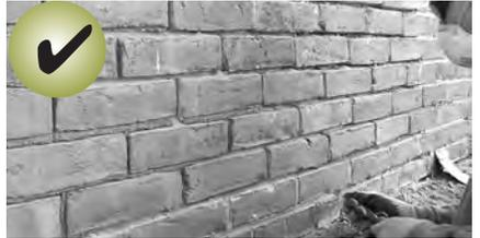
*Repoint mortar joints where there is evidence of deterioration. Commence with building cleaning again after any repointing has completely cured.*
