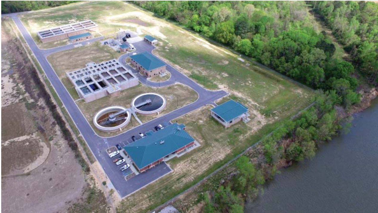
CAMDEN WASTEWATER TREATMENT FACILITY
